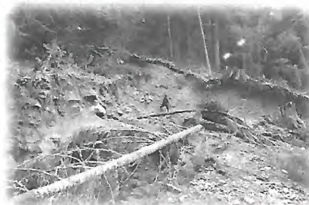
Washout along Mountain Loop Highway
