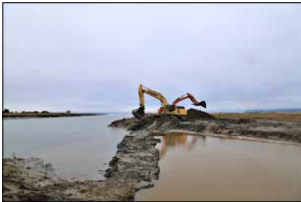
Leque Island Dike Removal
